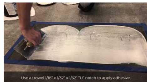
Use a trowel 1/16" x 1/32" x 1/32" "U" notch to apply adhesive.
